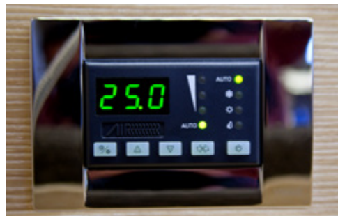
Air condition (up to 32.000 BTU) 3 units
