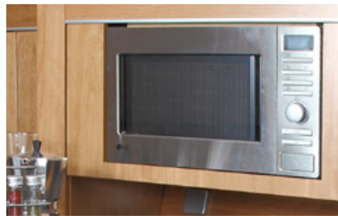
Flush installed microwave in galley
