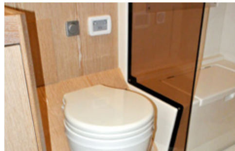
Electric toilet with sea water flush
