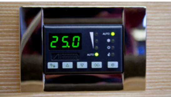
Air condition (32,000 BTU) with 4 outlets
